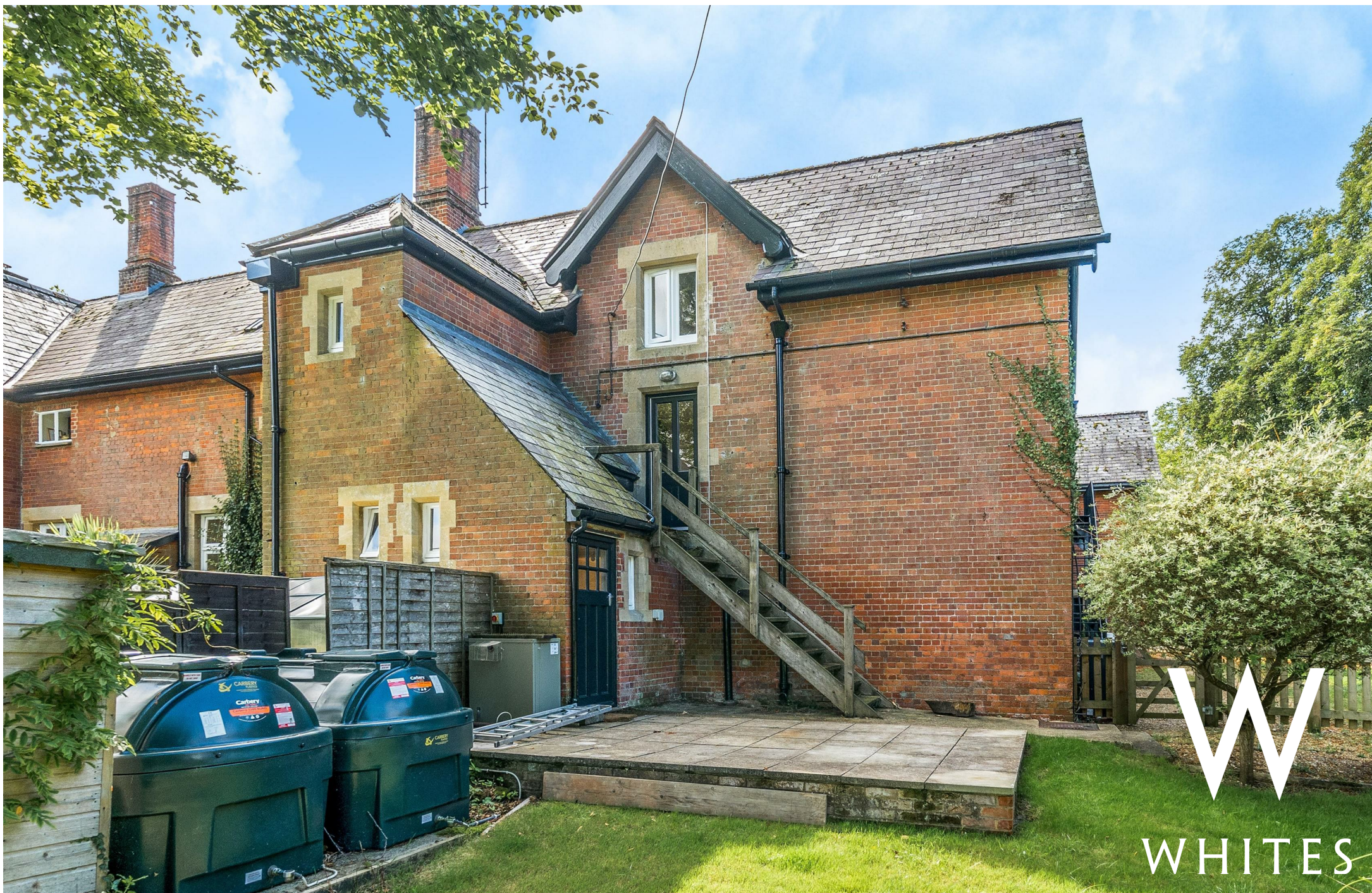
Stables Flat, 84 Longford Park, Bodenham, Salisbury, Wiltshire, SP5 4EG
